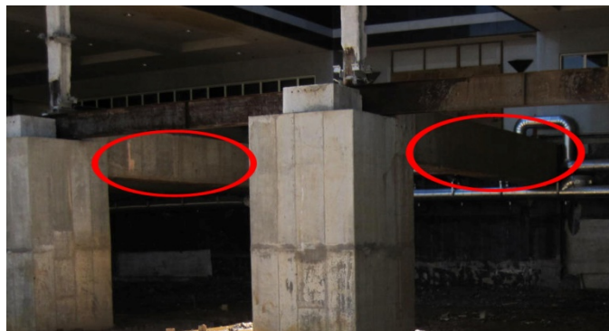
IMAGE 4: Existing Grade Beams
